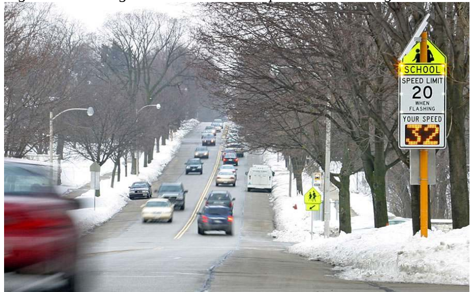
Figure 2: Flashing Beacon with Radar Speed Feedback Sign
